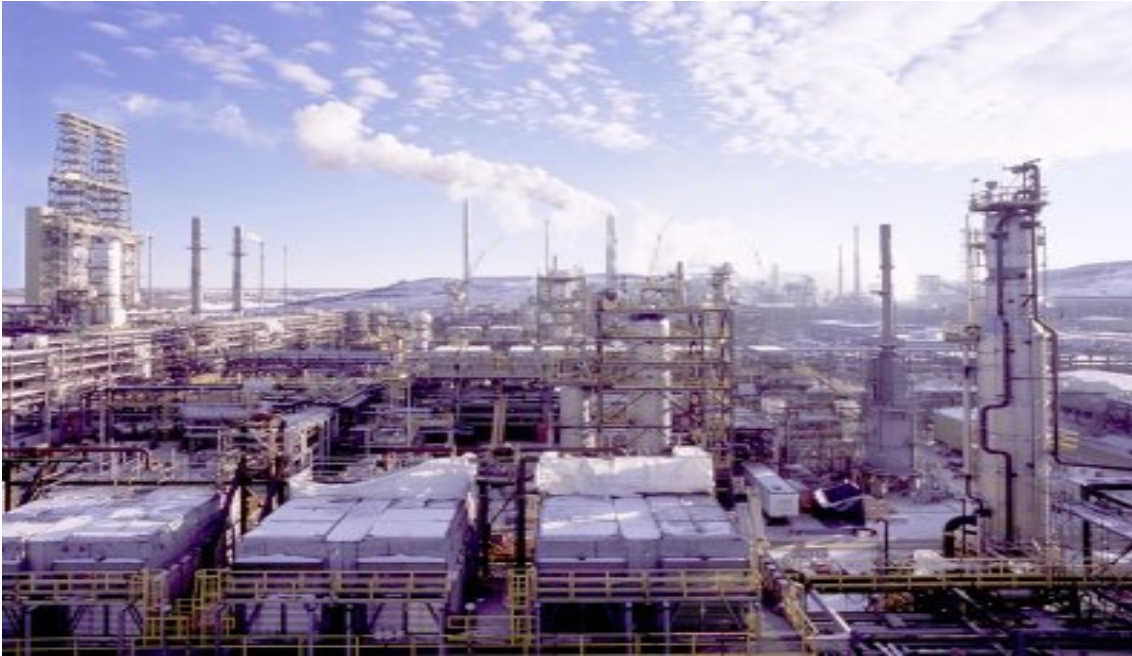
Figure 1 Suncor Energy, Inc. Upgrader Facility, Fort McMurray, Canada
